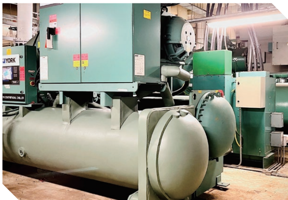
As part of the AI chiller plant optimisation system, we have installed new chiller plant systems with energy saving features. 作為人工智能冷水機組優化系統的一部分，我們安裝了具有節能功能的新冷水機組系統。
