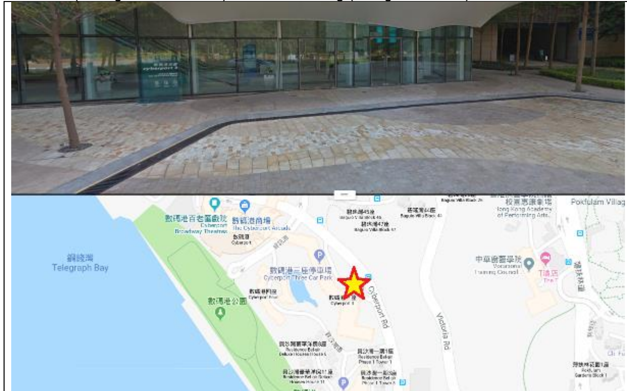
Drop-off area at Core E, Cyberport 3
